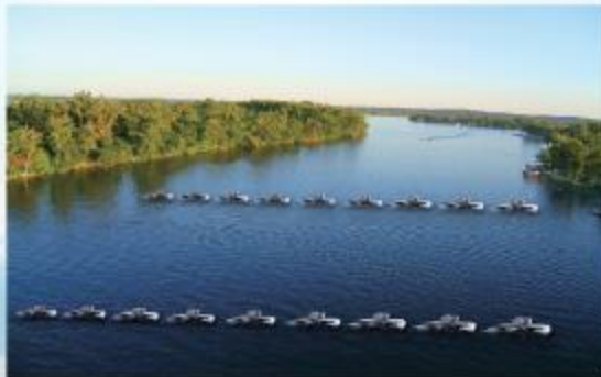
Floating type hydropower generator in series connection
